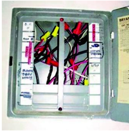
Breakers keep tripping so let's take it out
