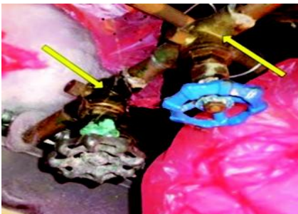
The first one couldn't shut off the water so let's put in a second one
