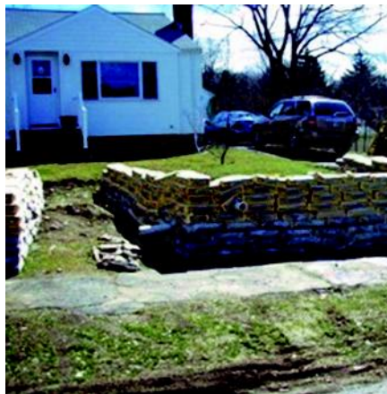
Eventually it will become a concrete wall equipped with weeping holes?
