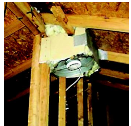
How to install an attic vent fan.....you require the following parts: drywall, sheet metal, fiberglass batt, wire ties, electrical tape, duct tape and nails
