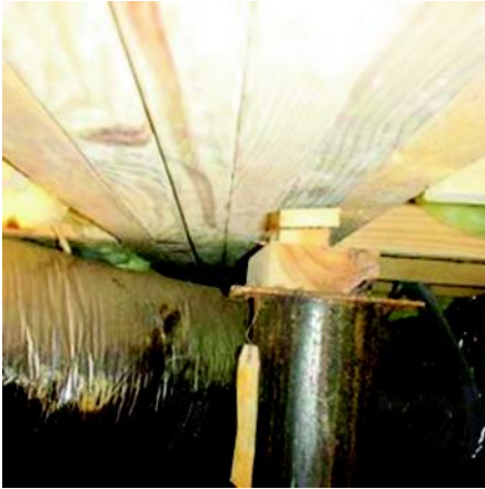
Off by a few inches, just use a couple pieces of wood to hold up the main joist
